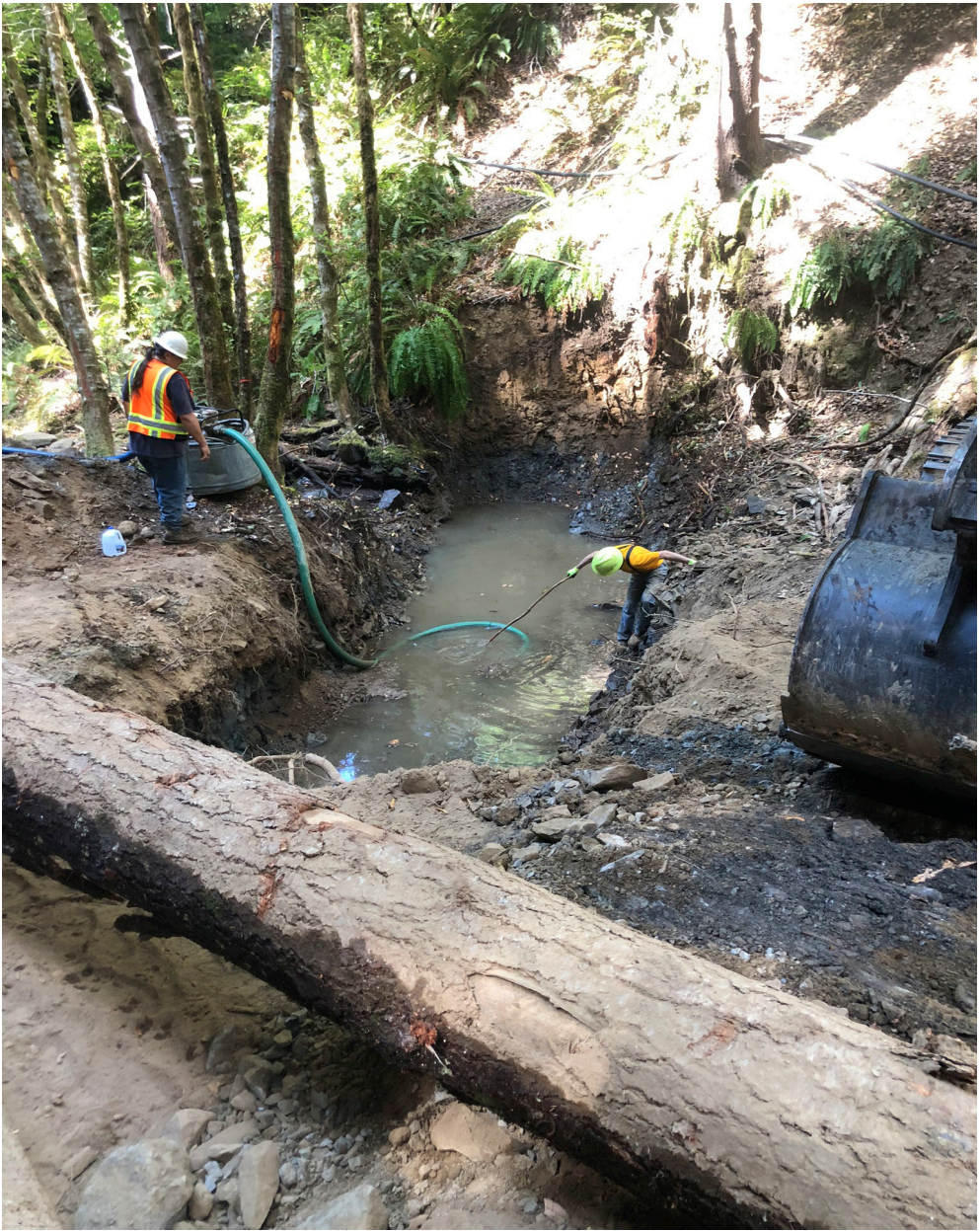
Above: De-watering the site at McKee Creek in preparation to construct a log weir. Photograph courtesy of Sanctuary Forest, Inc.
